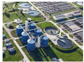
Waste & Sewage Treatment
