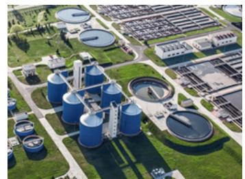
Waste & Sewage Treatment
