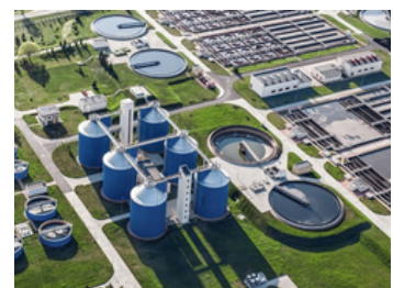
Waste & Sewage Treatment
